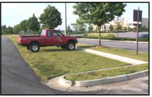
Figure 28: Grass Paver Used for Parking (Source: Georgia Stormwater Manual, 2001)
