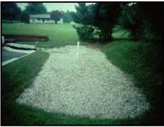
Figure 39: Infiltration Trench (Source: MA EOEA, 2005)
