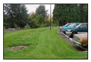
Figure 31: Use of a Grassed Filter Strip (Source: MA EOEA, 2005)
