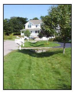
Figure 34: Another Example of an Open Vegetated Channel (Source: MA EOEA, 2005)
