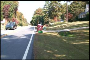
Figure 33: Examples of Open Vegetated Channels (Source: Georgia Stormwater Manual, 2001)
