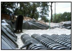
Figure 40: Infiltration Chambers (Source: MA EOEA, 2005)
