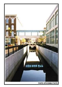
Figure 46: Daylighting Arcadia Creek in an Urban Area in Kalamazoo, MI (Source: Stormwater Magazine, Nov/Dec 2001)
