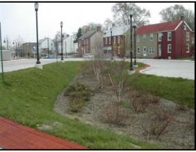
Figure 36: Example of a Bioretention Facility Along Roadway
