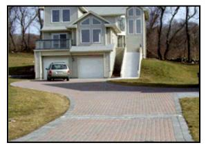
Figure 20: Permeable Pavers as an Alternative Driveway Surface (Source: MA EOEA, 2005)
