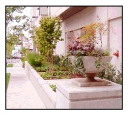
Figure 43: Stormwater Planters (Source: MA EOEA, 2005)
